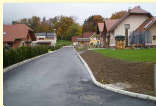
The new road section at the community hall Dobrovlje
