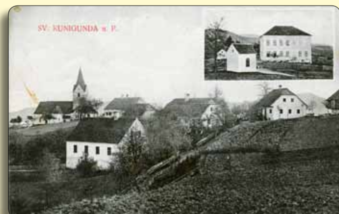
Gorenje – the former primary school
