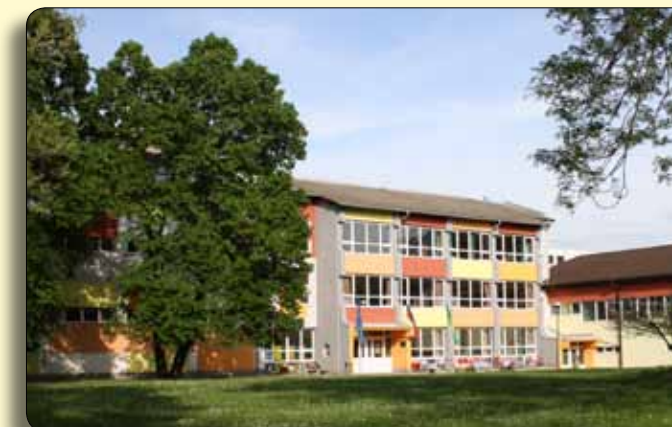
Renovated primary school in Zreče
