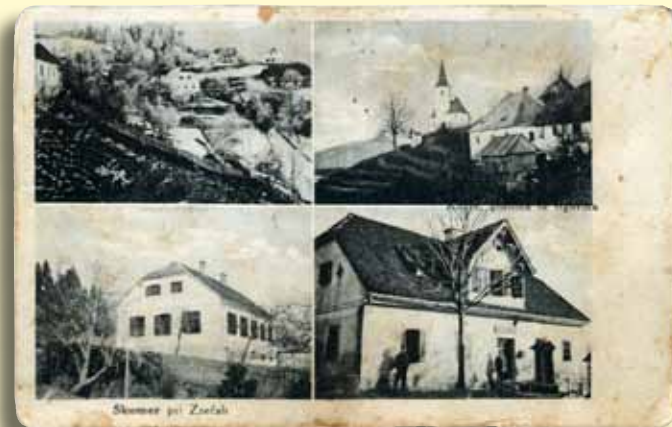
Skomarje – school building bottom left
